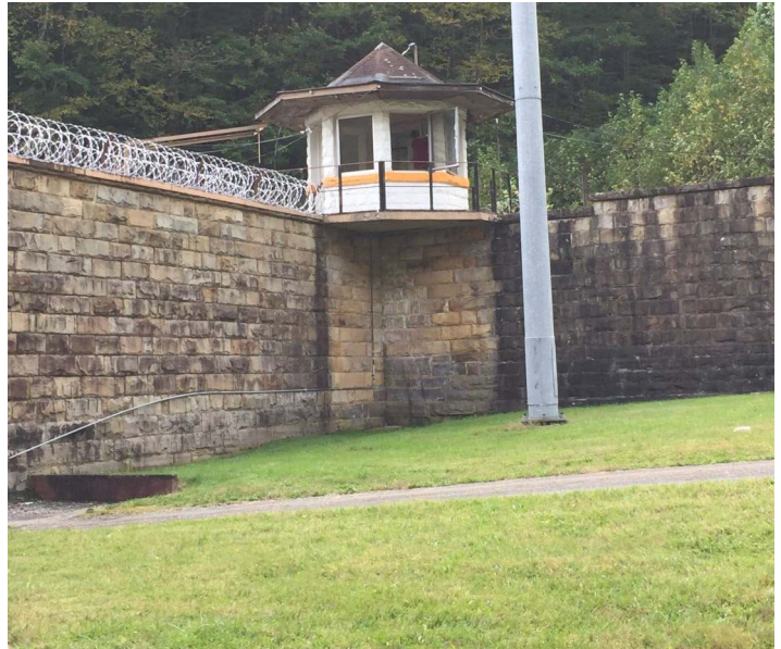
Guard towers are located in the corners of the prison yard.
